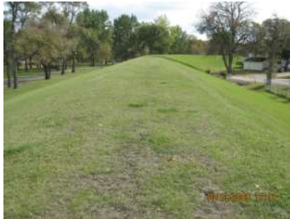
Near 6 th Ave. S. & 3 rd St. S. in Fargo, ND Height: 15 ft, Side Slopes 1:3
