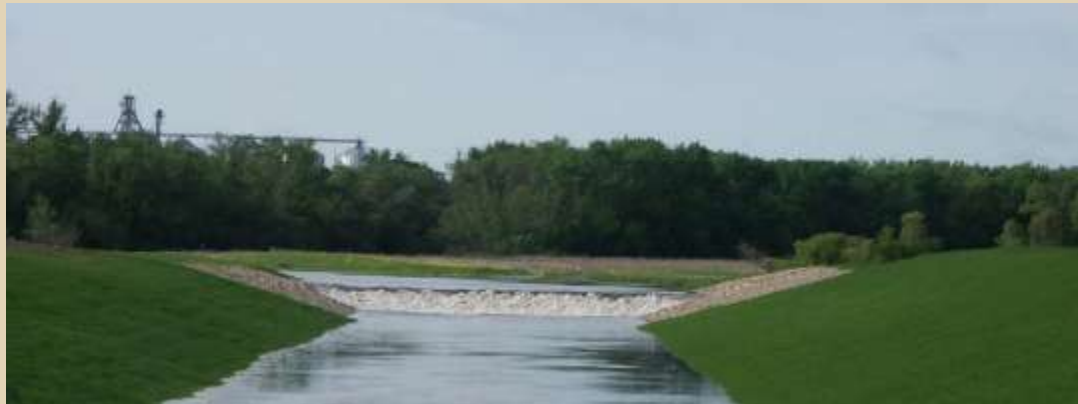
Fixed weir at Breckenridge, MN Diversion
